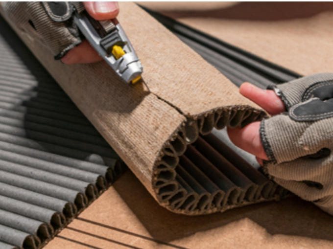
Step 1: Use a hooked knife blade to carefully add a relief cut through the backing material only, this will allow a single rib to stretch.
